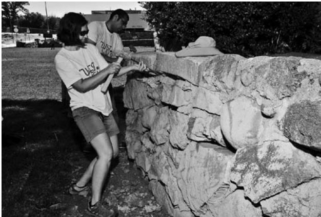
Barrie Schuster, one of the organizers of West of Wells, works to remove old mortar in preparation for repairing of the old rock wall at Stewart Park. Photo courtesy of Susan Mantle.
