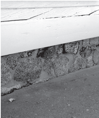
Mortar repairs to the Truckee River rock foundation (left) and to the brick porch pedestal (right) give this old beauty at 524 Holcomb a fresh look with the same character as the original materials. Photos by Char Eckmeyer.
