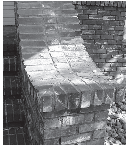
Mortar repairs to the Truckee River rock foundation (left) and to the brick porch pedestal (right) give this old beauty at 524 Holcomb a fresh look with the same character as the original materials. Photos by Char Eckmeyer.
