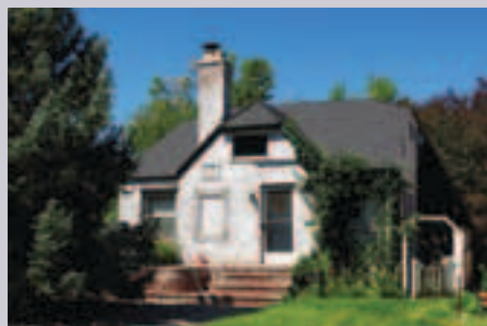
This house, located at 1015 Gordon, illustrates a cross-gabled roof with a twist: the gable peaks are clipped, resulting in a jerkinhead shape.
