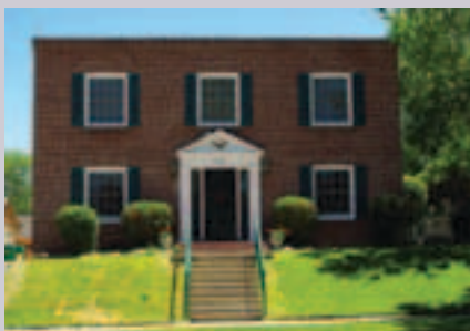
832 Nixon Avenue has a flat roof with parapet.
