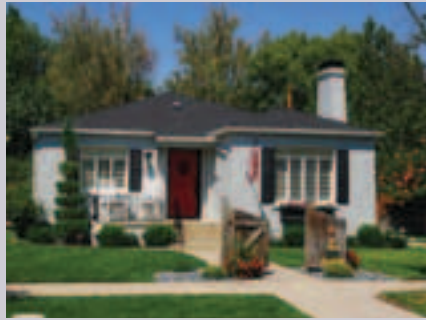
1031 Manor's roof is an example of a cross-hipped pyramidal roof.
