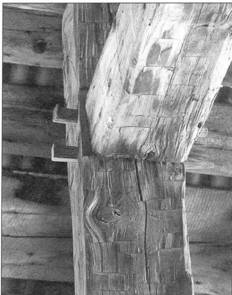
Hand-hewn beams joined together by a mortice and tenon joint with wooden pins.
