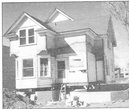
Front of 93 Bell, 1988. The Bevilacqua movers raised the home up on blocks and a block foundation was built under it. The new foundation extends out on the right where an addition to the house was built.
