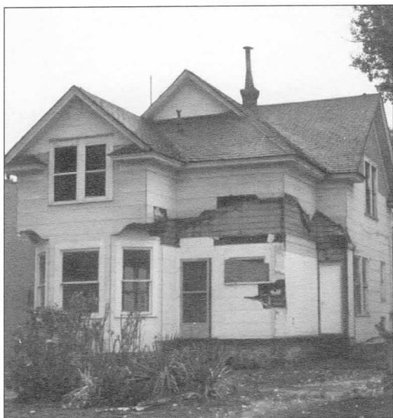
The front of 93 Bell in 1987. There was originally an L-shaped porch on the right of the house but they had neglected to put a foundation beneath it, so it was sagging and unsalvageable.
