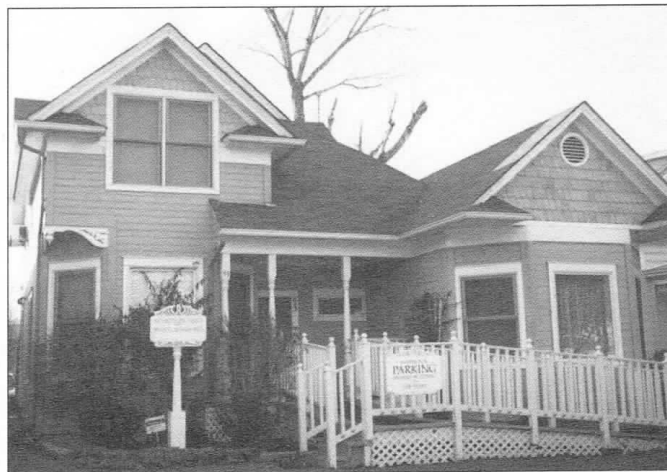
The renovated 93 Bell in 1989. A new block foundation was installed under the house and extended out to the right where a one-story addition to the house was built. Photos courtesy of the Atchesons.
