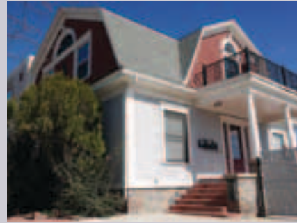
820 N. Center is one of Reno's best examples of a cross-gambrel roof.
